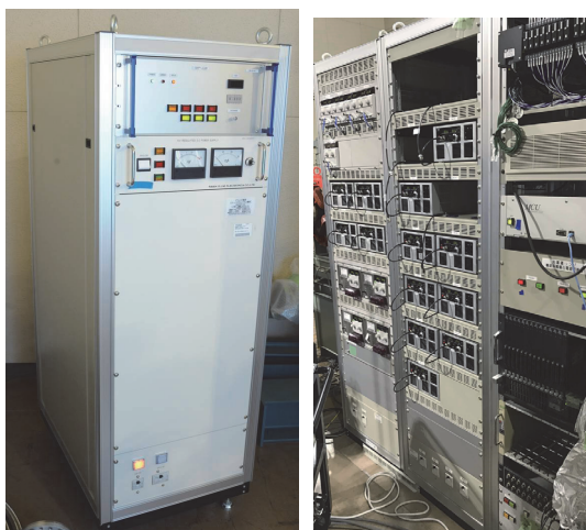
Fig. 3 New power supplies for the extraction septum at the booster synchrotron (left) and those for the beam transport line magnets (right).
